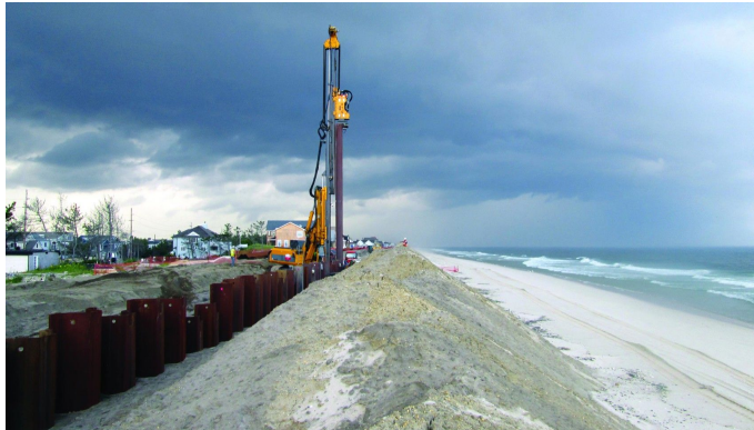
Sea wall in NJ installed after Hurricane Sandy, Mott Macdonald 2014
