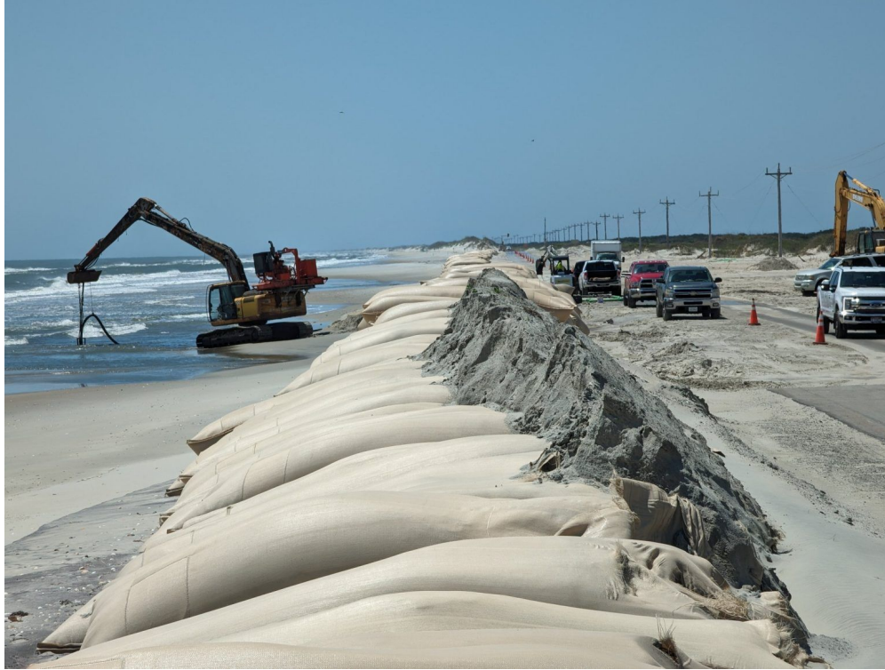
Sand bagging along breached dune on Ocracoke Island NCDOT 2025
