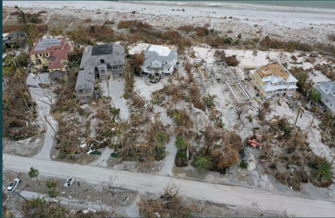
Hurricane Ian damaged nearly every structure on Sanibel 1
